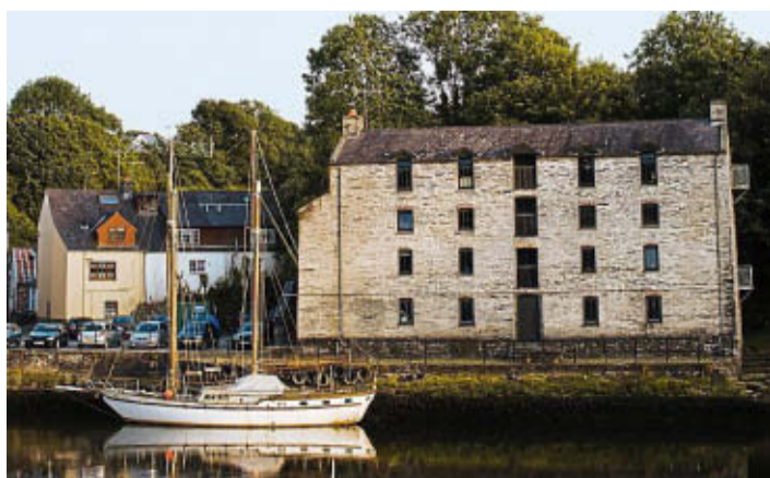
Two warehouses have been converted into The Albion in Aberteifi
